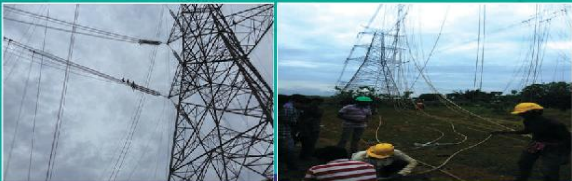
765 KV Erection at Gurla mandal, vizianagaram District.
