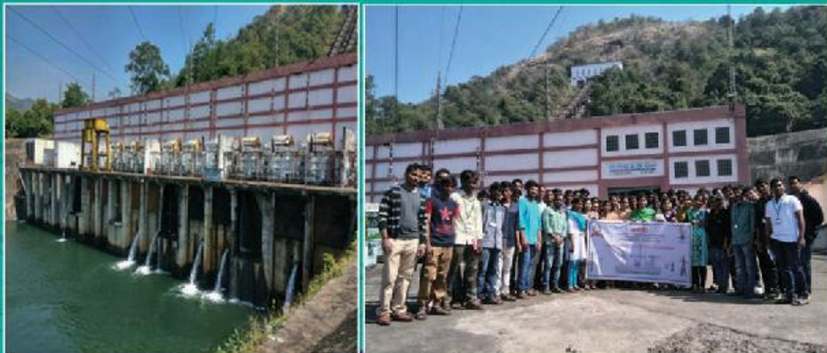
Lower Sileru Hydro Electric Power House, APGENCO
